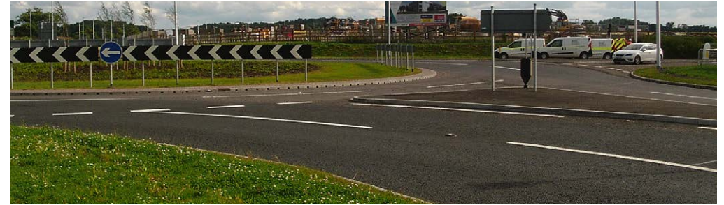
Worcester Six highway works
